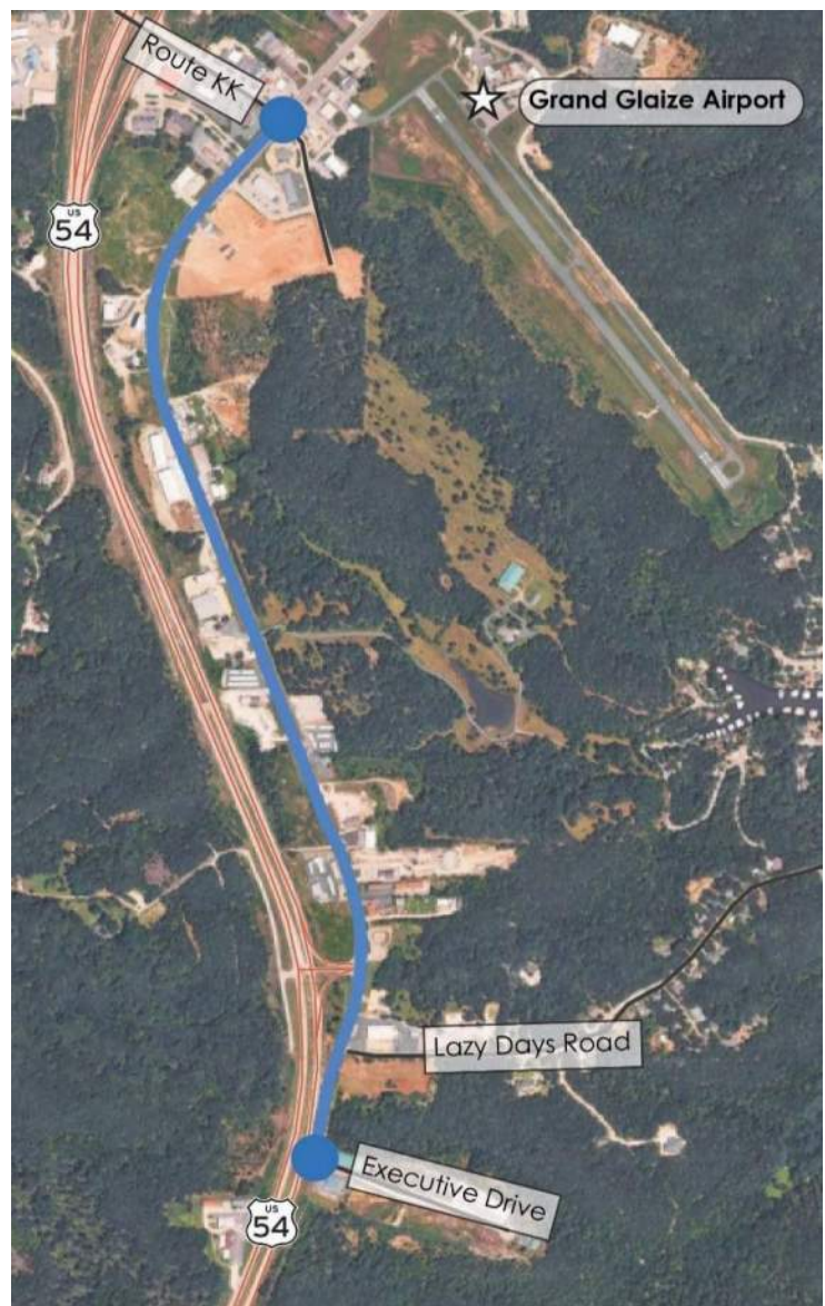
Figure 89 - Aerial image of Osage Beach Parkway Segment 1: Executive Drive to Route KK
