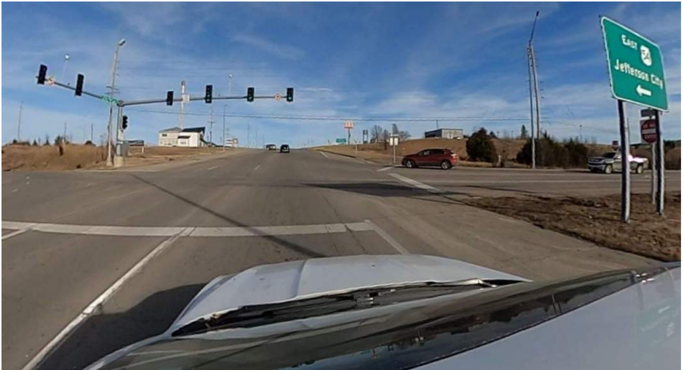
Figure 62 - Pedestrian Accommodation EB Osage Beach Parkway NB U.S. 54 Ramp Terminal (02.11.2026)
