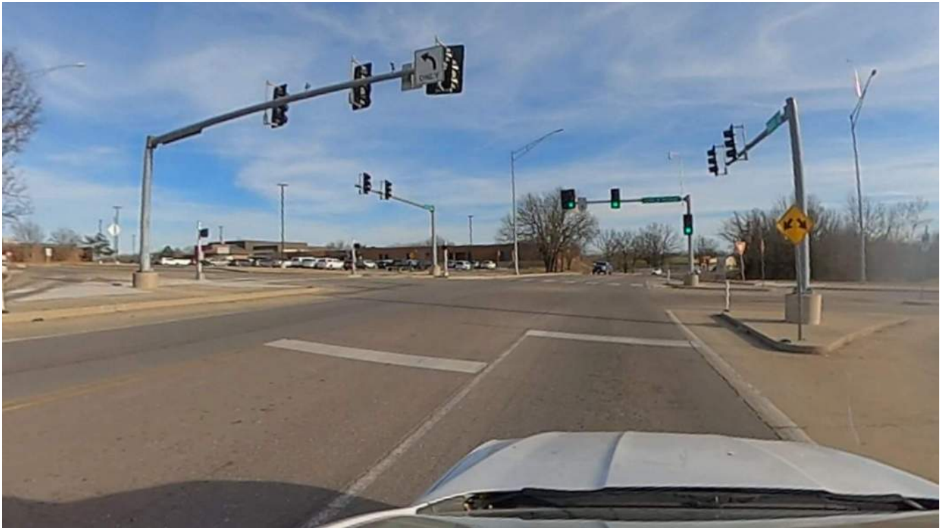
Figure 110 - Facing Southbound on Route 42 (Photo taken 2/11/2026)
