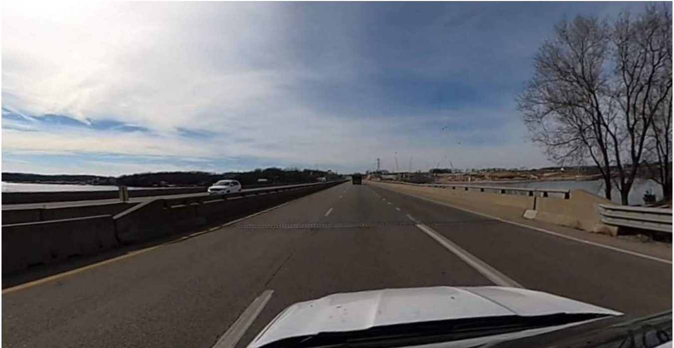
Figure 4 - Westbound Grand Glaize Bridge (02.11.2026)
