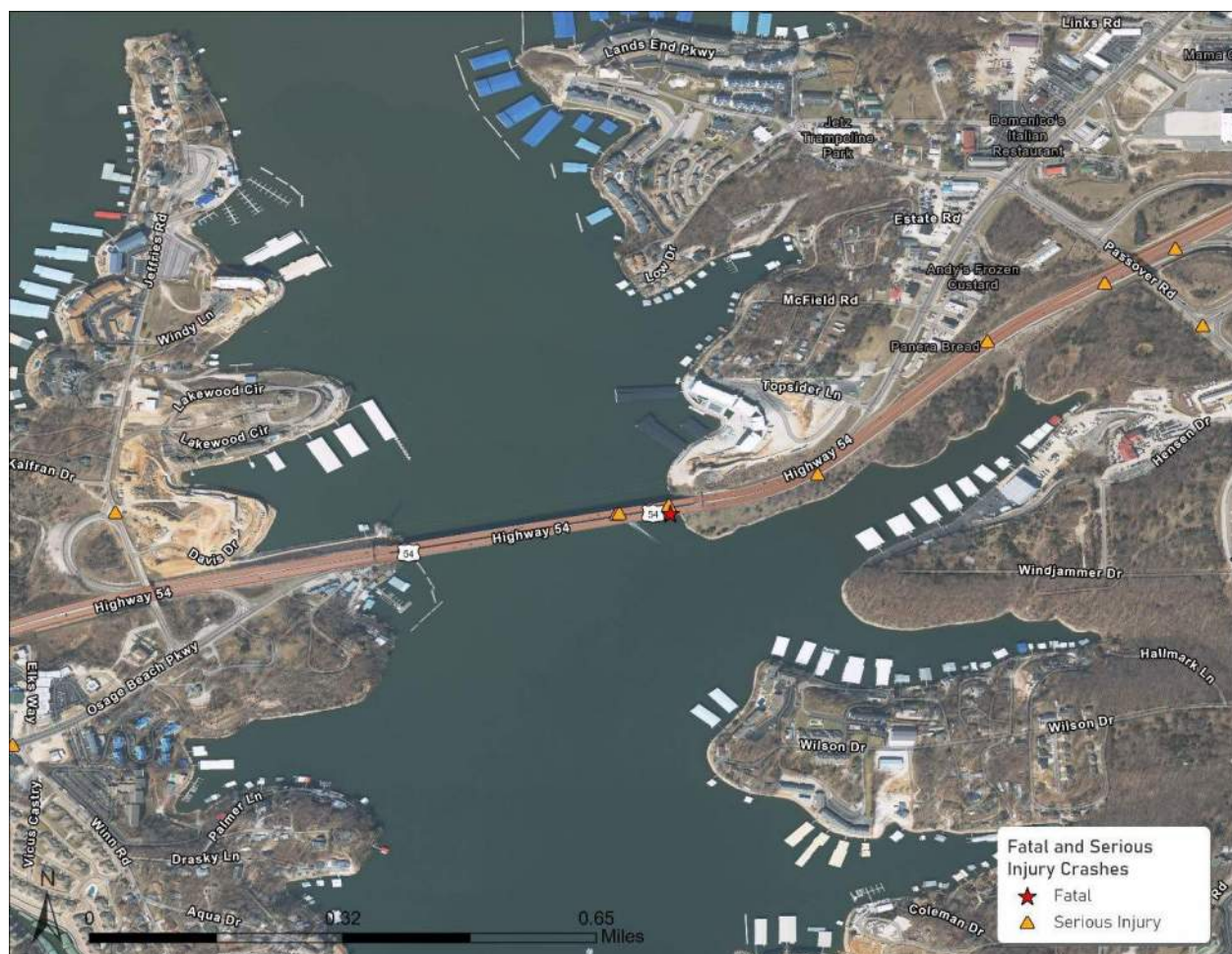
Figure 18 - Grand Glaize Bridge Aerial with Fatal and Serious Injury Crashes 2020-2024
