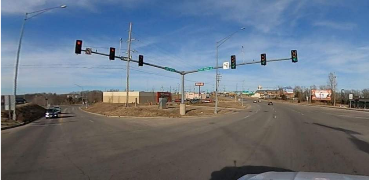
Figure 74 - Pedestrian Accommodation Eastbound Osage Beach Parkway & Fort Osage Lane (02.11.2026)
