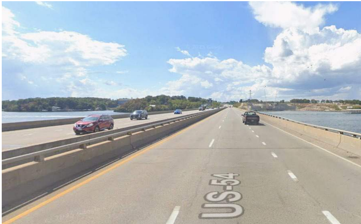
Figure 19 - Grand Glaize Bridge Facing Westbound
