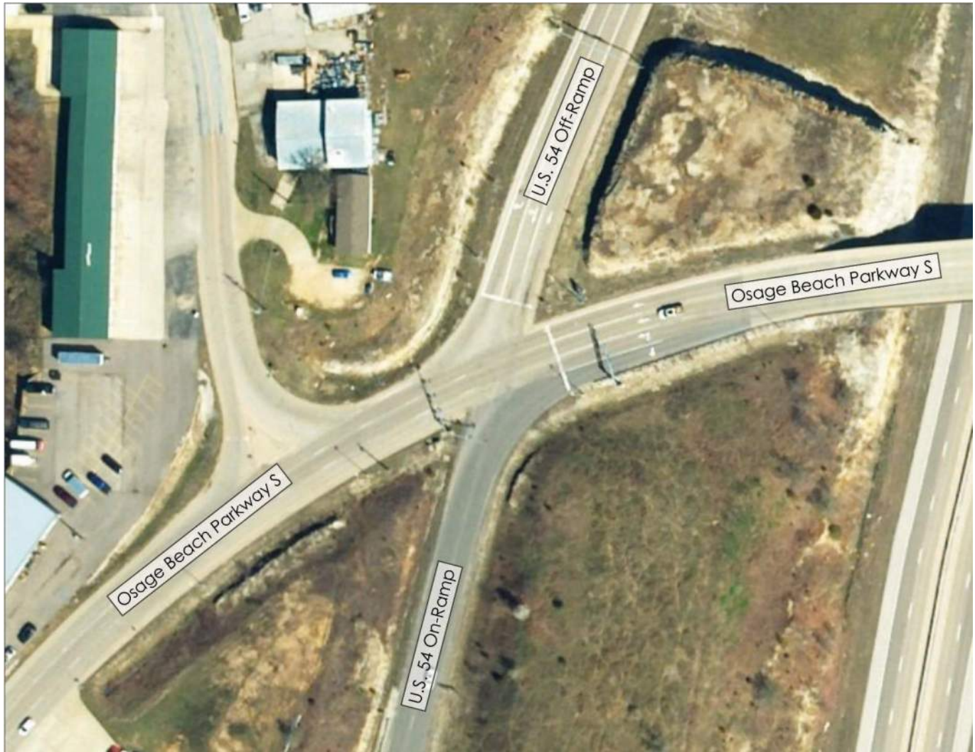
Figure 65 - Aerial image of the Osage Beach Parkway & WB U.S. 54 Ramp Terminals
