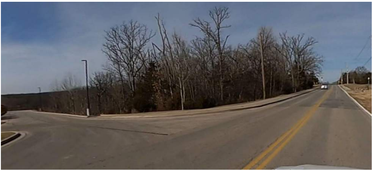
Figure 116 - Sidewalk infrastructure north of Nichols Road (02.11.2026)
